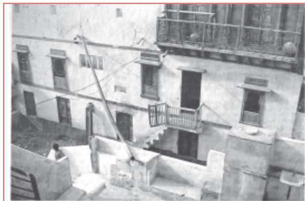
Rooftop harvesting was common across the towns and villages of the Thar. Rainwater that falls on the sloping roofs of houses is taken through a pipe into an underground tanka (circular holes in the ground), built in the main house or in the courtyard. The picture above shows water being form a neighbour's roof through a long pipe. Here the neighbour's rooftop has been used for collection of rainwater. The picture shows a hole through which rainwater flows down into an underground tanka .
